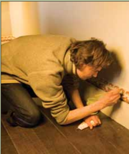
Applying "size" to the skirting board so that the gold leaf will stick
