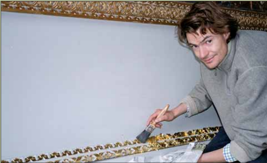
Rupert Coke skewing off the excess gold leaf from a skirting board
